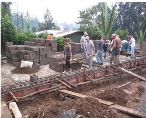
Annie & Dan Wilson helping to build daycare center
